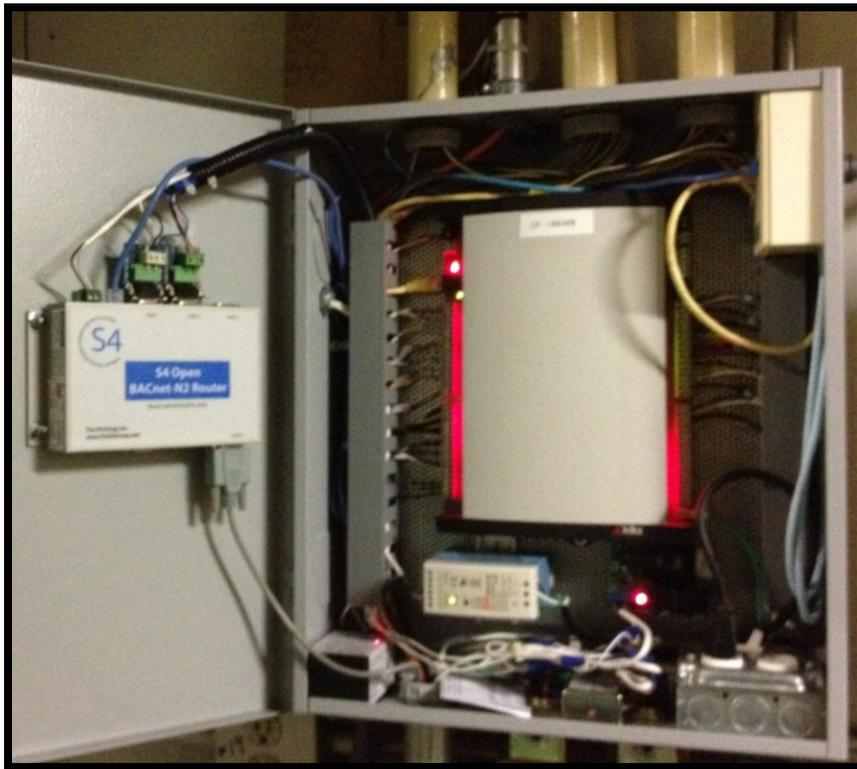
ENTEC chose the S4 Open: BACnet-N2 Router as the best solution for this project. The installation was quite simple. The BACnet-N2 Router was installed utilizing the Upstream N2 Interface transparently providing co-existence with the legacy Metasys® head end system. Utilizing this unique S4 Open appliance capability eliminated the need to remove or disconnect any of the Metasys® head end hardware.
